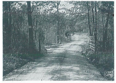
Turn out bars on roads keep erosion at a minimum.
