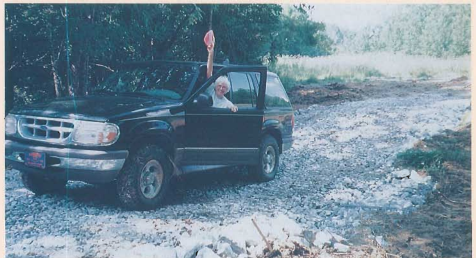
Completed wire basket crossing ready for traffic.
