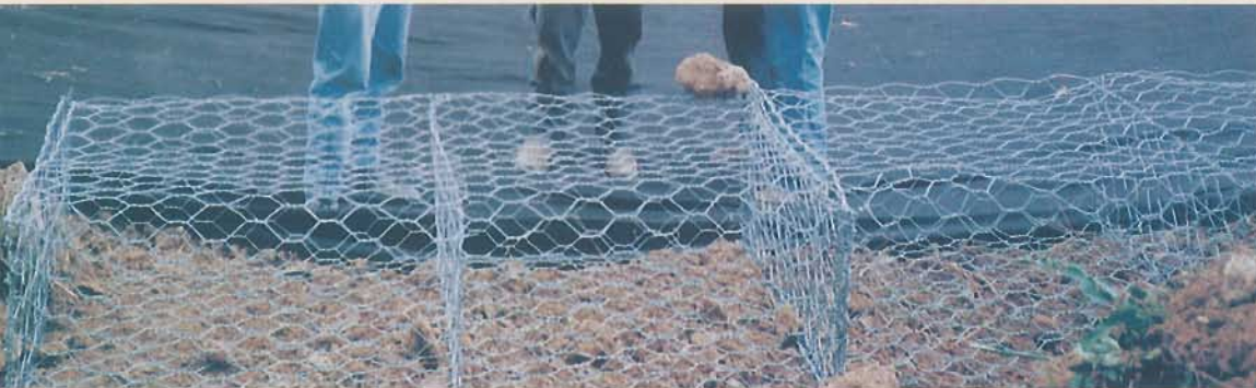
The assembled gabion wire basket.
