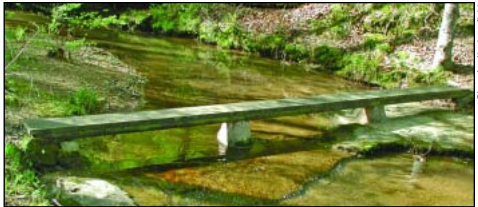
An acrylic concrete additive in this simple footbridge makes pedestals more durable and helps them set better and stronger.
