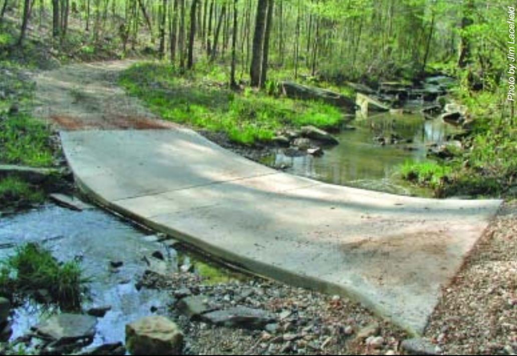
This curved low-water bridge contains three small culverts that allow normal flows to pass beneath the surface of the bridge, which remains dry 95% or more of the year.
