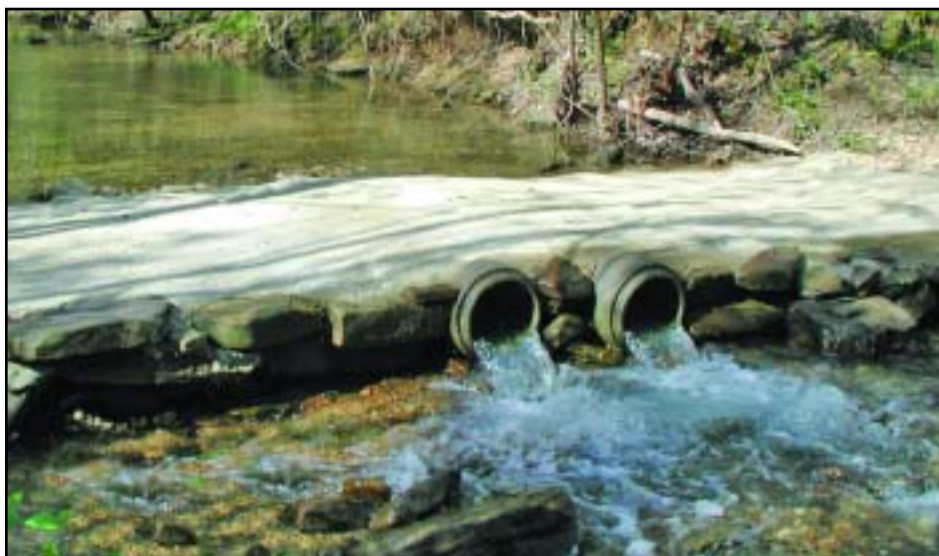
Concrete culverts are a mainstay of forest trail construction and with a little imagination, they easily blend into natural surroundings.
