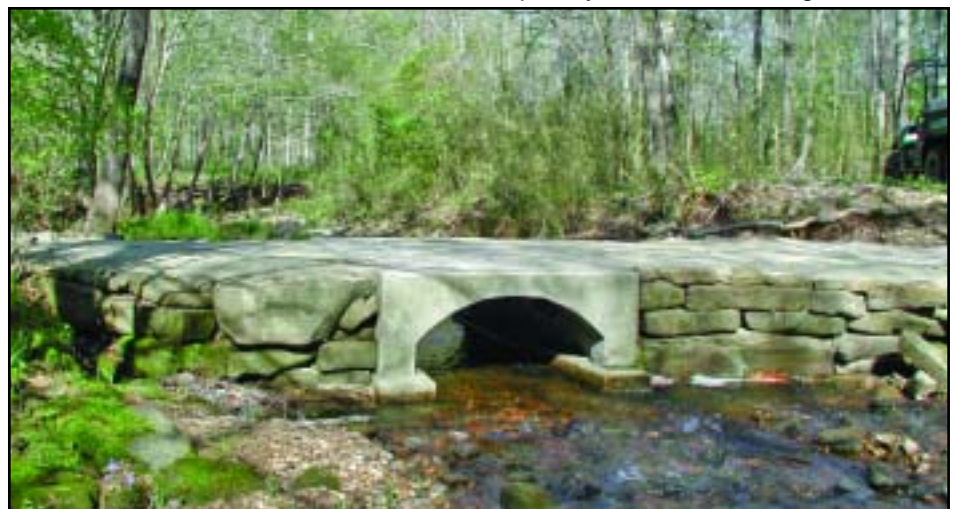
These low-water bridges still allow most flood water to pass over the top, but are raised up higher from the streambed to accommodate steeper banks.
