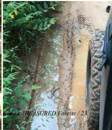
Mud is a warning sign of poor drainage and maintenance ahead.
