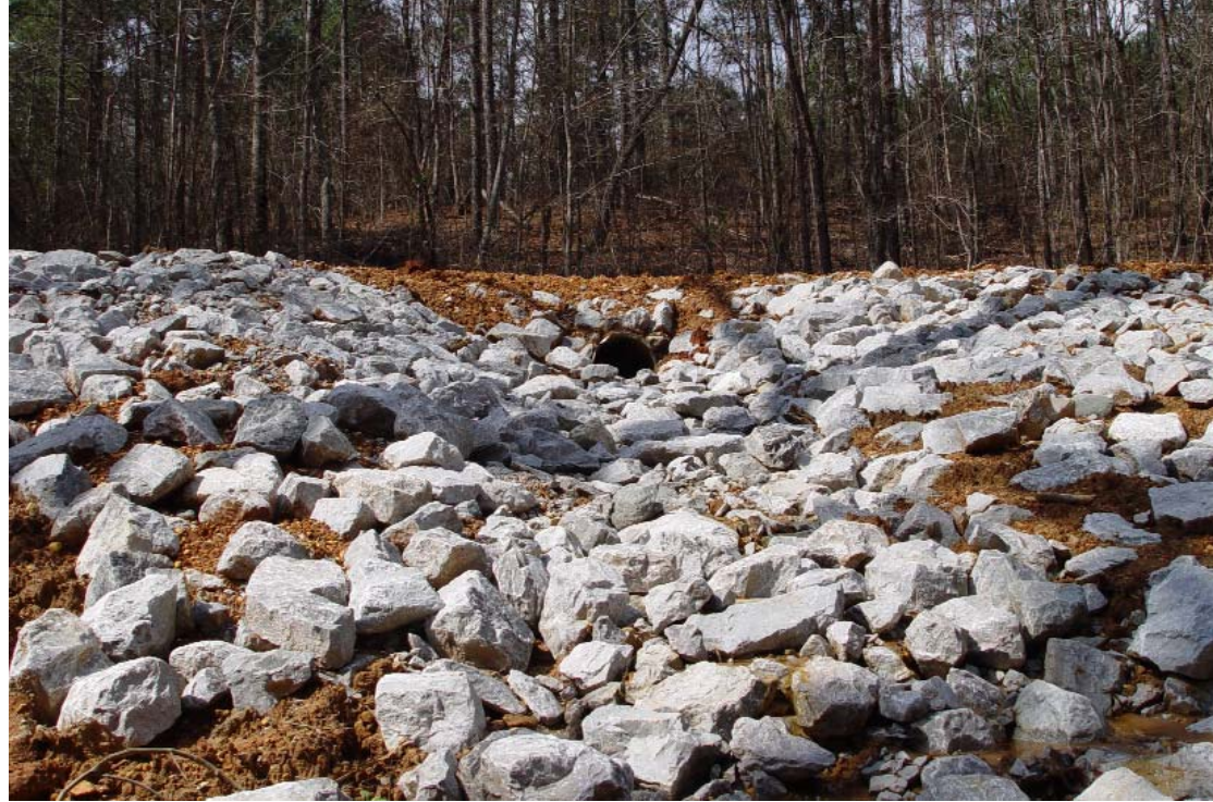
Proper culvert installation.
