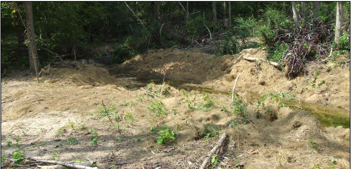
Cleared stream crossing, stabilized with hay.
