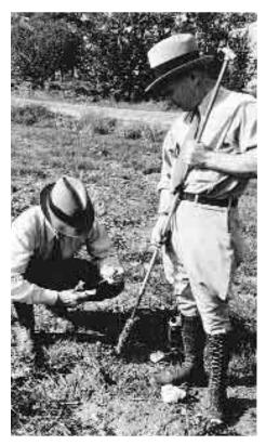
The screw auger was the primary tool used by the soil scientist in the early days. Texturing by hand was one of the first "soil tests" and continues to be a tool for the soil scientist today.
